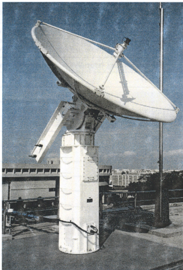
Fig 2: Photograph of the installed 3-meter dish for the Singapore radar system.
