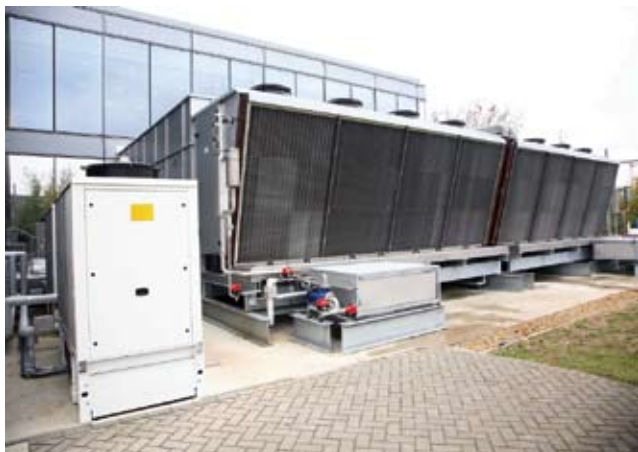
Figure 3 External view of a typical free cooling module. Photograph provided courtesy of Keysource ( www.keysources.co.uk ).
