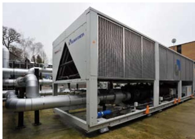
Figure 2 One of ECMWF's Turbocor based chillers.
